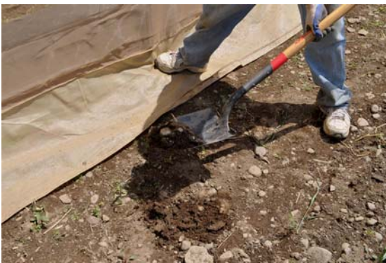
11. The bottom flap is buried to hold down the fabric and seal the cage.
