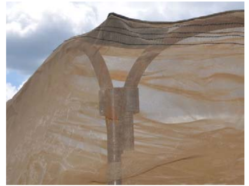
10. The life of the fabric is extended by inserting padding where it contacts pipe junctions.
